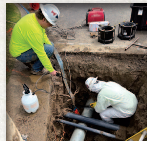
NESSWD crew working on water line repair.
