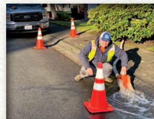
Flushing a water line.
