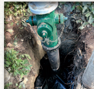
Completed installation of new fire hydrant.
